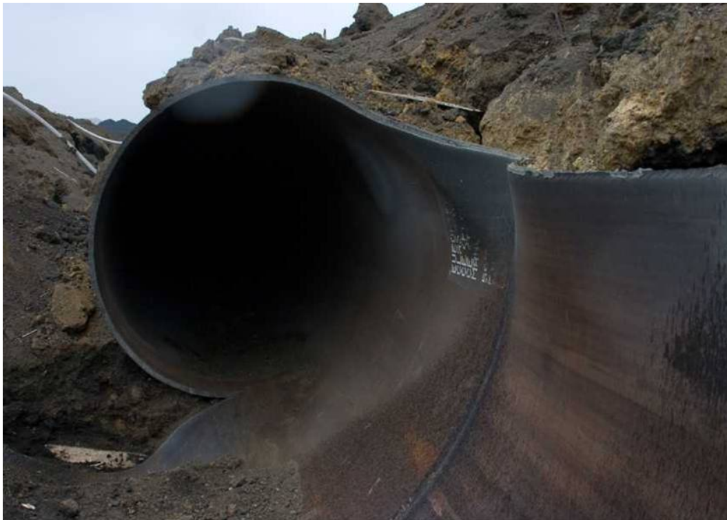
Figure 18: Crack Arrest after full scale test
